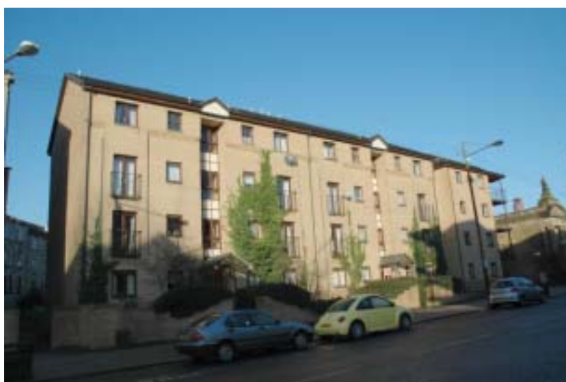
St George's Road block at St George's X, Glasgow
